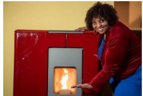
The open fireplace in the Ngewanas' lounge was replaced with a [Calore Piazzetta](#) closed-combustion pellet fireplace. With the warmth from the fire and new insulation, the Ngewana family never needed their electric heaters this winter and greatly reduced their use of the gas heater.
