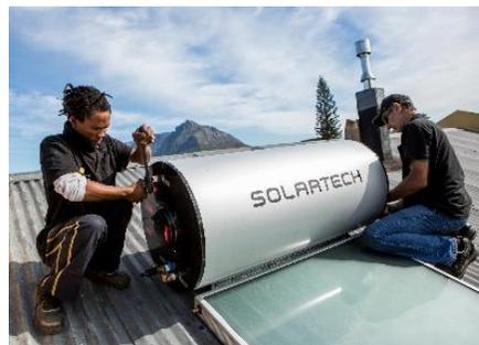
The solar water heater was sponsored and installed by [SolarTech](#), but would have cost about R28 000 after a R9 000 Eskom rebate advanced by the installer. That expense would have been covered by savings within 4 to 6 years, a normal range for a family of four or more. The system carries a 10 year warranty.
