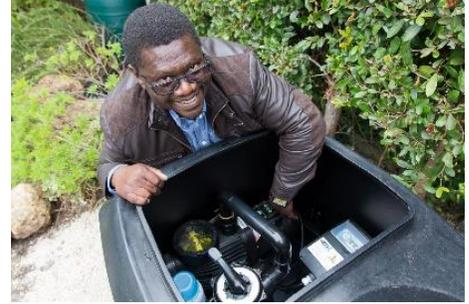
The Ngewanas' old pump was one of the largest users of energy in the house. The combination of reduced hours and a new [Speck Badu Eco Touch variable-speed pump](#) has made this one of the most dramatic improvements in efficiency at the Ngewana household. Compared to their old pump running 10½ hours a day, they will save about R3 500 in the coming year.
